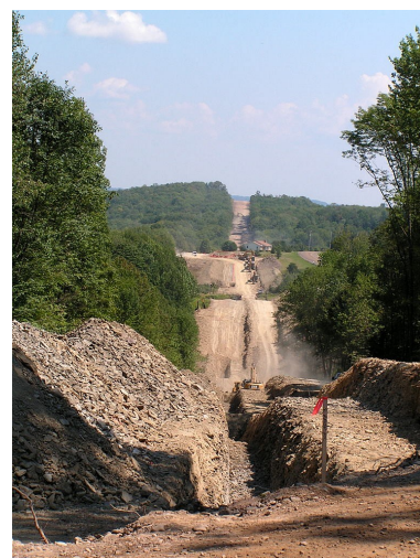
Photo of the Millennium Pipeline crossing Germany Hill on August 24, 2008
